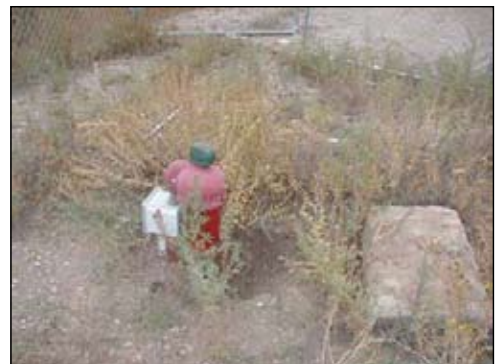
Another example of an unprotected wellhead.
