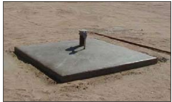
Example of a properly protected wellhead.
